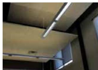
properties of the hemp hurd, a suitable application for this material is as an aesthetic ceiling tile. The tiles are formed by bonding a "slurry" of hurd and adhesive or resin under elevated heat and pressure.
